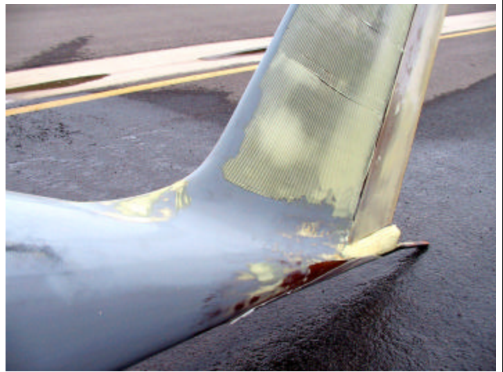
This not only shows the vertical stabilizer faring, but also the notched trowel method of applying micro. The white spots are where the surface was low.
